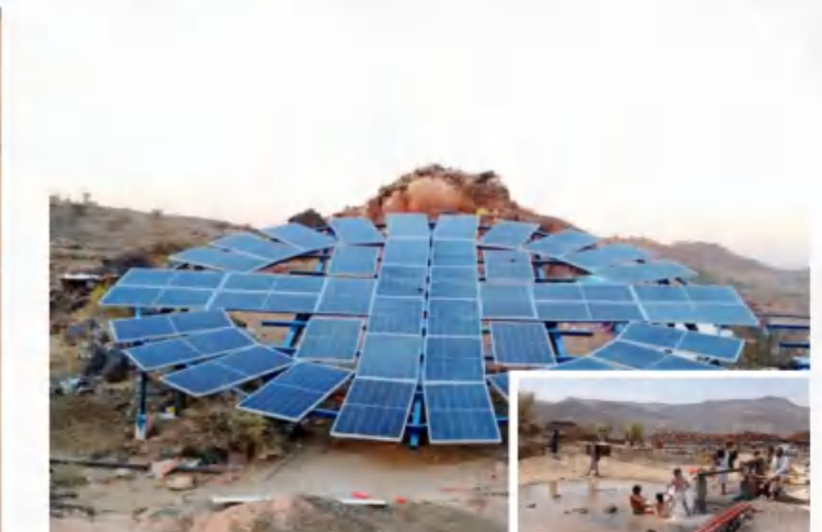
55kW Solar pumping System
