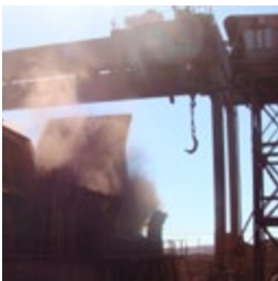
Crane Control Demanding application at South African mine
